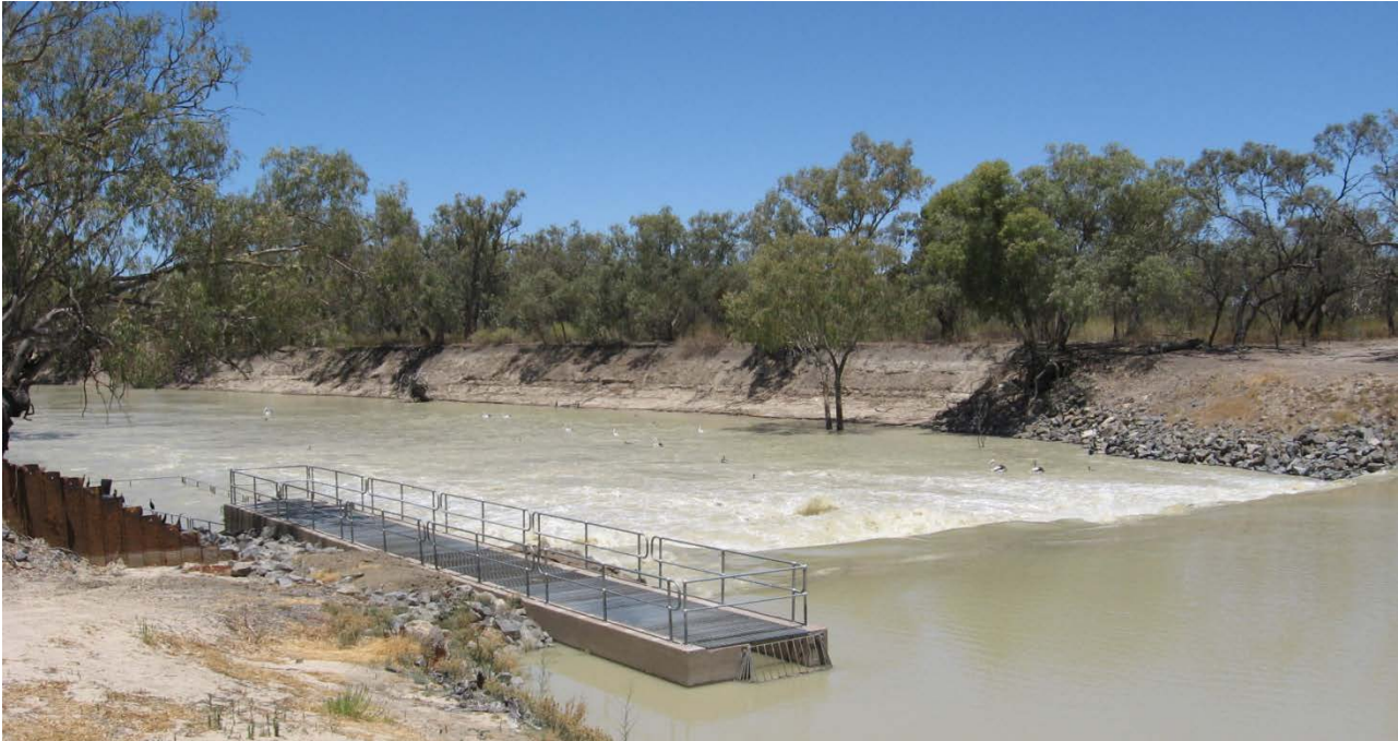
Figure 1 – Increased releases from the Menindee Lakes have taken the flow at Weir 32 above 3,000 ML/day. The upper part of the fish ladder can be seen in the foreground.
