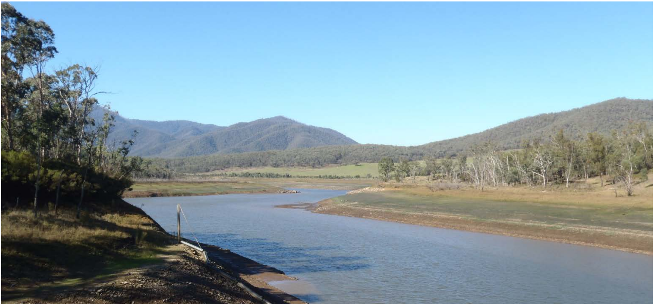
Photo 1 – The regulating pondage downstream of Dartmouth Reservoir was lowered during the week, prior to the current high flows, for maintenance works (Photo courtesy: Peter Liepkalns, Goulburn-Murray Water)
