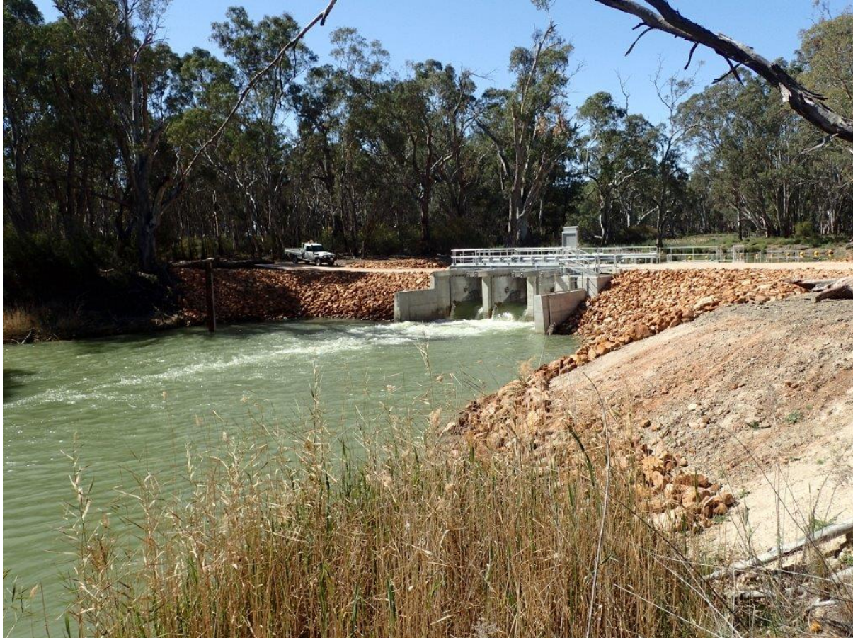
Photo 1 – The new Mullaroo offtake that manages flows into Mullaroo creek. The new regulator includes a fishway providing fish passage between the renowned Murray Cod habitat of Mullaroo creek and the River Murray. The fishway has been constructed to help increase populations of this iconic fish (Photo by Allan Drechsler, 31 August 2015).
