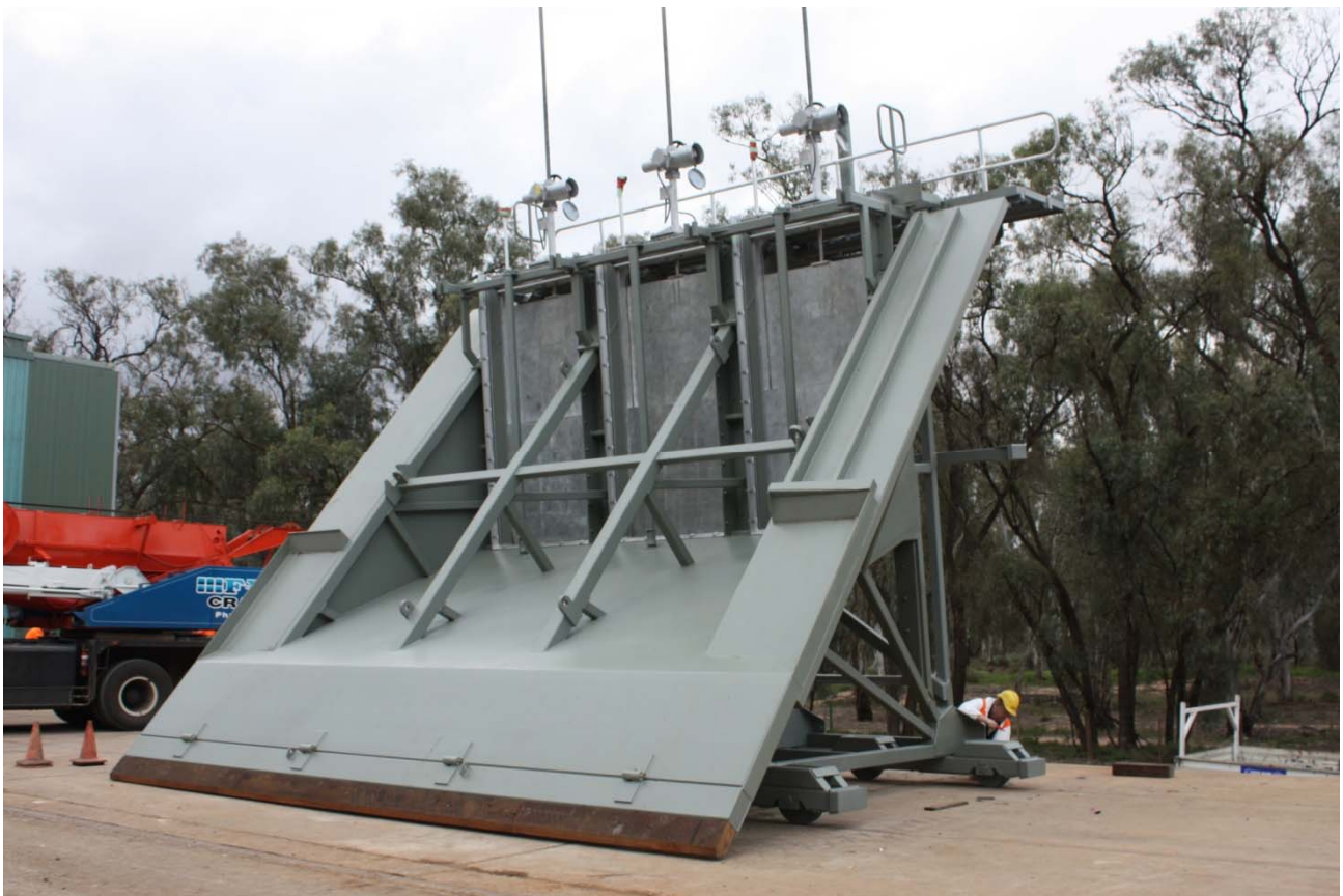
Figure 1 Mildura Weir trestle - pre-installation (Source: Phil Pfeiffer MDBA)
