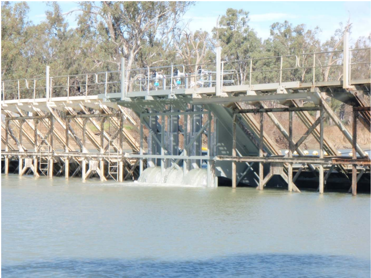
Figure 2 Installed Trestle at Mildura Weir (Source: John Prentice MDBA)
