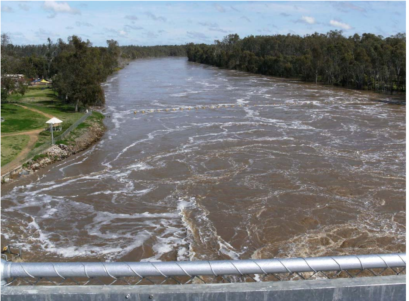
Figure 2 Flood waters flow downstream of Yarrawonga Weir on the River Murray, 8 th September 2010. Photos: Pat Doyle, Goulburn-Murray Water
