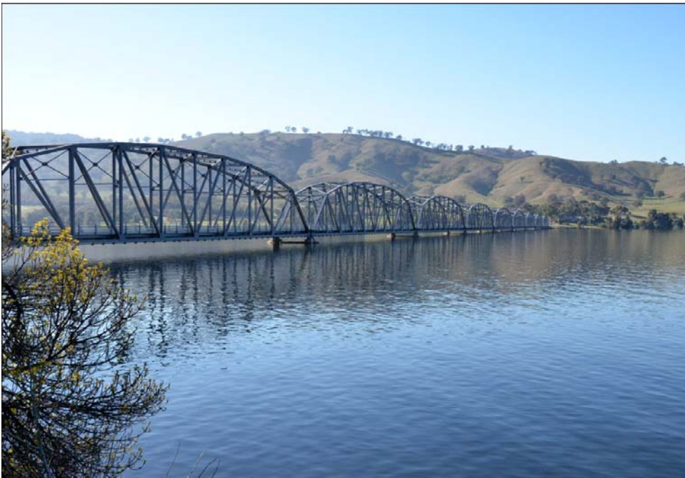
Figure 1 - The Bethanga Bridge at Hume Reservoir on 15 September 2011: one day after regulated releases began. Photo: Andrew Bishop, MDBA
