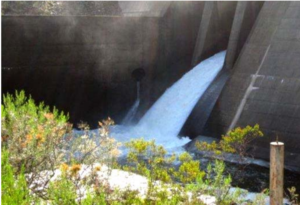
Figure 1 – Riparian flow of 200 ML/day released to the Mitta Mitta River from the regulating pond downstream of Dartmouth Reservoir on 21 February 2012 (Photo courtesy Catherine Goonan, MDBA)
